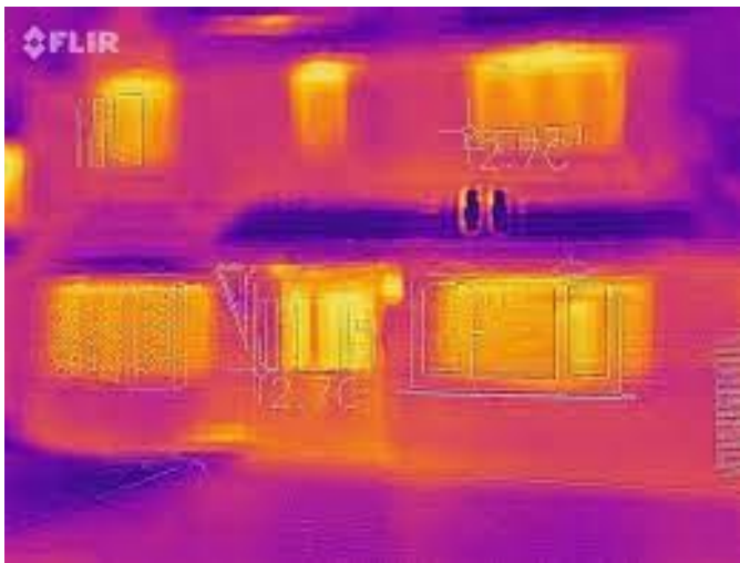
Image: octopus.energy. Viewing a house through the thermal imaging camera.
